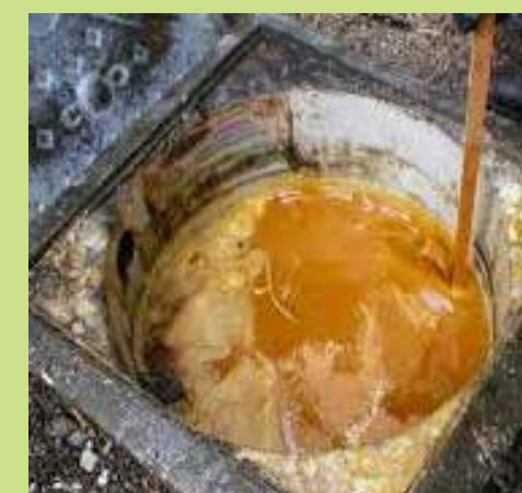
If you do, the hot fat will turn solid when it hits cold pipes and end up blocking your drains (as shown in this photo, taken on a call-out to one of our homes).
